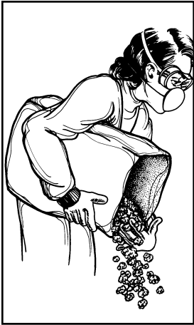
Figure 2: Wear protective clothing when installing insulation.
