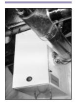
An air-to-air heat exchanger is a balanced ventilation system, meaning that it exhausts out and brings in an equal amount of air. Its heat recovery feature makes it one of the more energy efficient ventilation systems available. parts: the minimum round-the-clock ventilation amount and the supplemental amount needed for peak occupancy and special activities.
